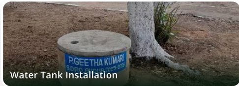
Water Tank Installation
