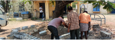
Apr 28 — Cattle trough work at the Veterinary Hospital
