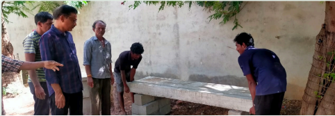
Jun 25 — Protective platform construction
